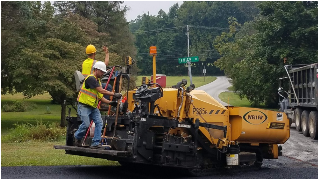
Township road paving project
