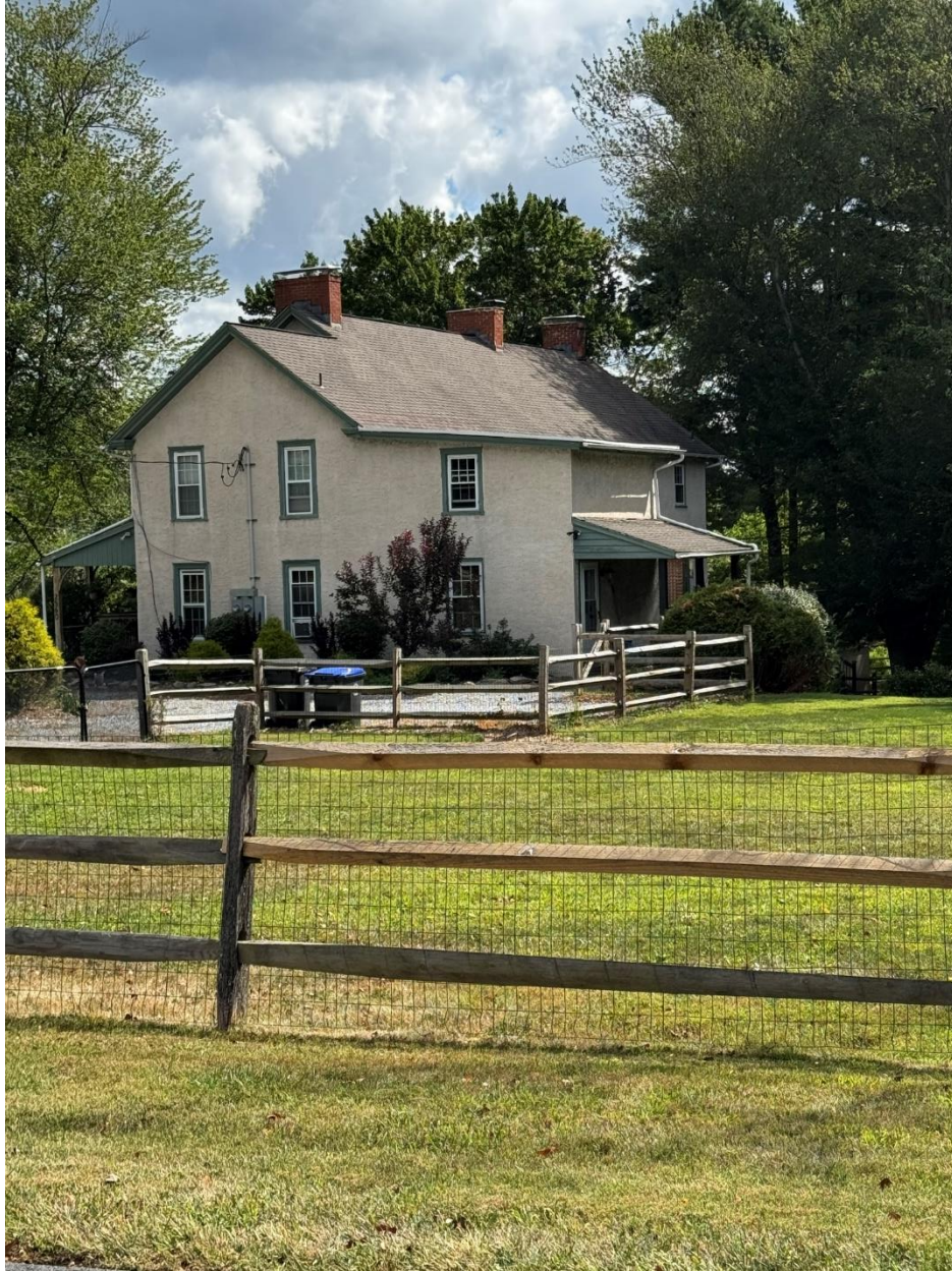
Elevation Looking Northeast - Photo taken 09/02/25
