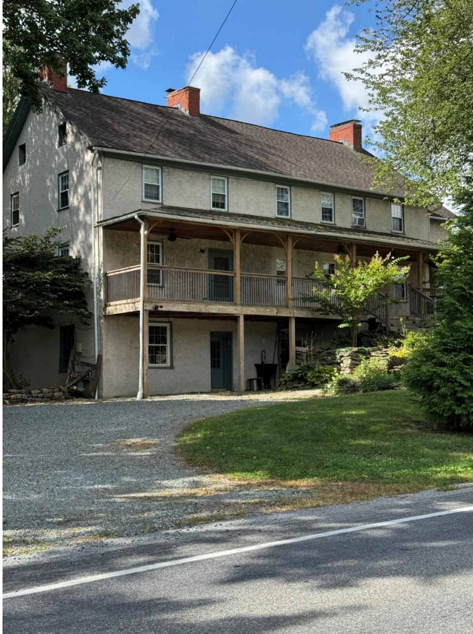
Elevation Looking South from Strasburg - Photo taken 09/02/25
