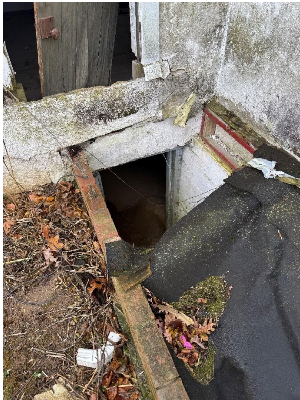
OPEN BASEMENT ENTRY
