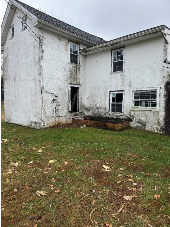
NORTHEAST PORTION (REAR) OF STRUCTURE
