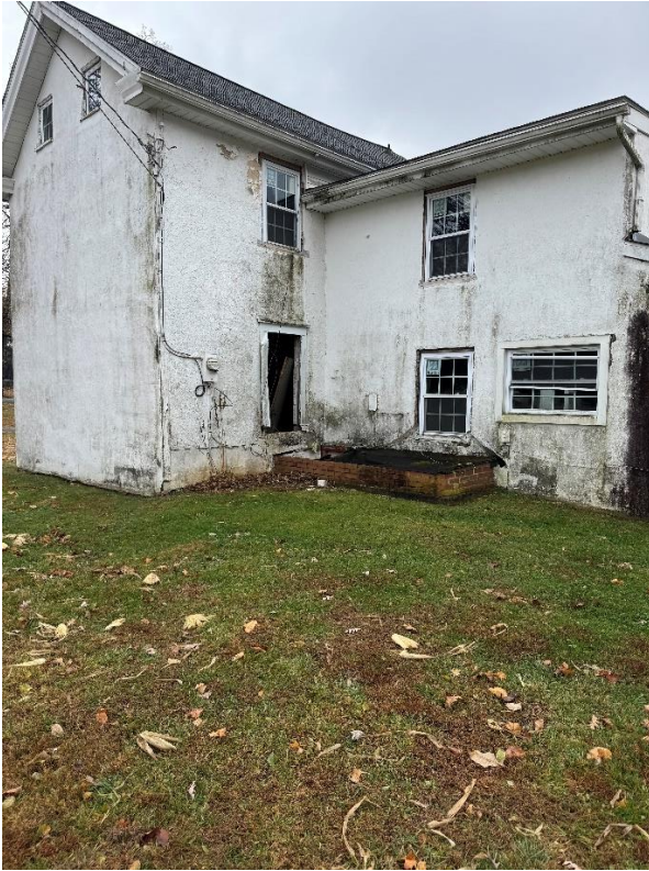
NORTHEAST PORTION (REAR) OF STRUCTURE
