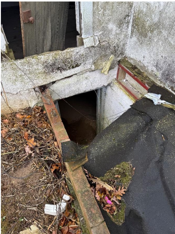
OPEN BASEMENT ENTRY
