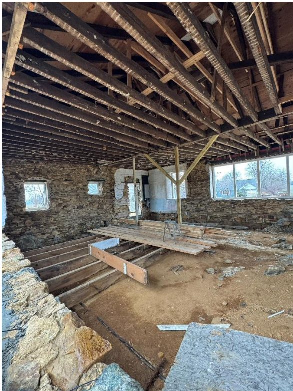
INTERIOR VIEW 03-04-2026 SURVEY 2965 STRASBURG ROAD
