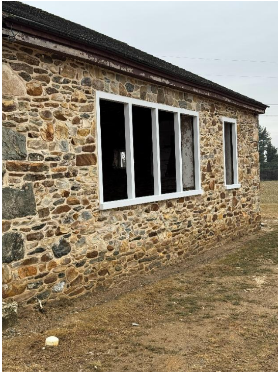
ELEVATION LOOKING EAST
